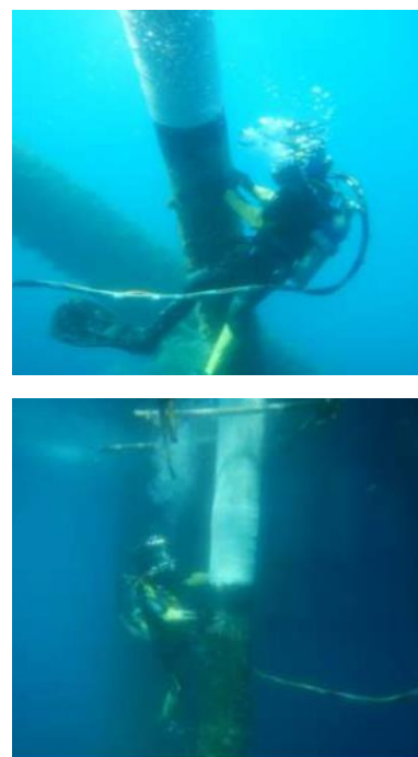
Figure 2.0: Condition of pipe after composite wrapping and top coat application.
