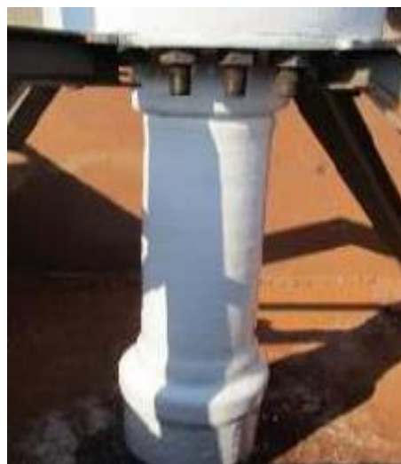
Figure 2: Image show the Xmas tree casing after wrapping application
