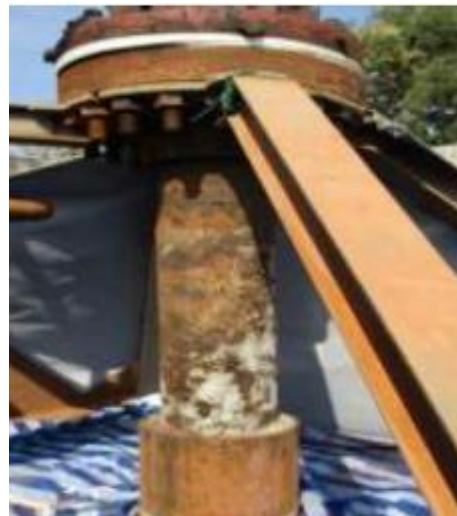
Figure 1: Image show the Xmas tree casing before wrapping application
