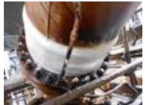
Figure 1.0: Condition of the leak prior to repair application
