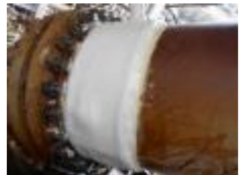
Figure 2.0: Condition of the pipe after wrapping and topcoat
