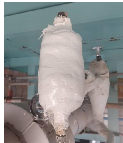
Figure 2.0: Condition of the pipe after wrapping and topcoat
