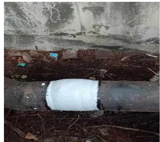
Figure 2.0: Condition of pipe after composite wrapping and top coat application
