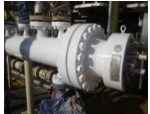
Figure 2.0: The appearance of 10" riser after applied with Corro-Chem™ 330 HHA
