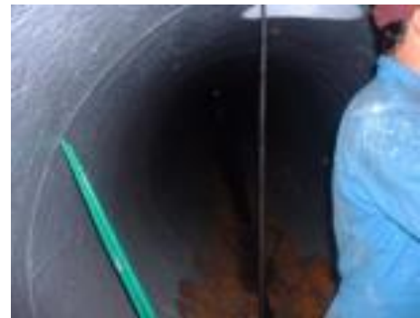
Figure 3.0: Applied Corro-Dur™ 258 over blasted surfaces
