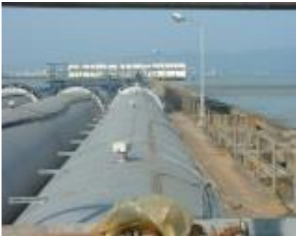
Figure 1.0: External view of the 500-meter pipeline
