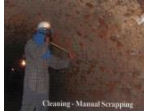
Figure 2.0: Manual scraping of barnacles and marine growth
