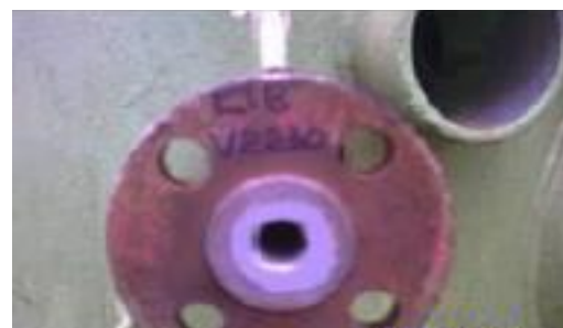
Figure 2: Application of Corro Dur 252 (Temperature <80°C)
