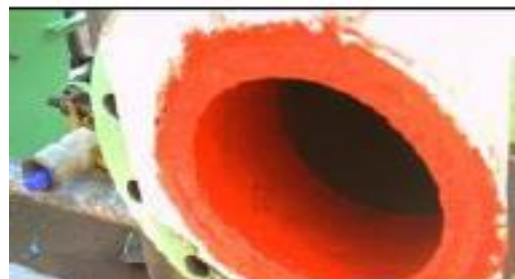
Figure 1: Application of Gas-Pruf 130 as primer
