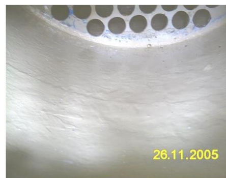
Figure 3: Compartment near the man way, fully top coated with Corro Chem 330
